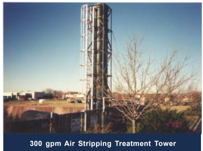
Tower Modification and Reconstruction
